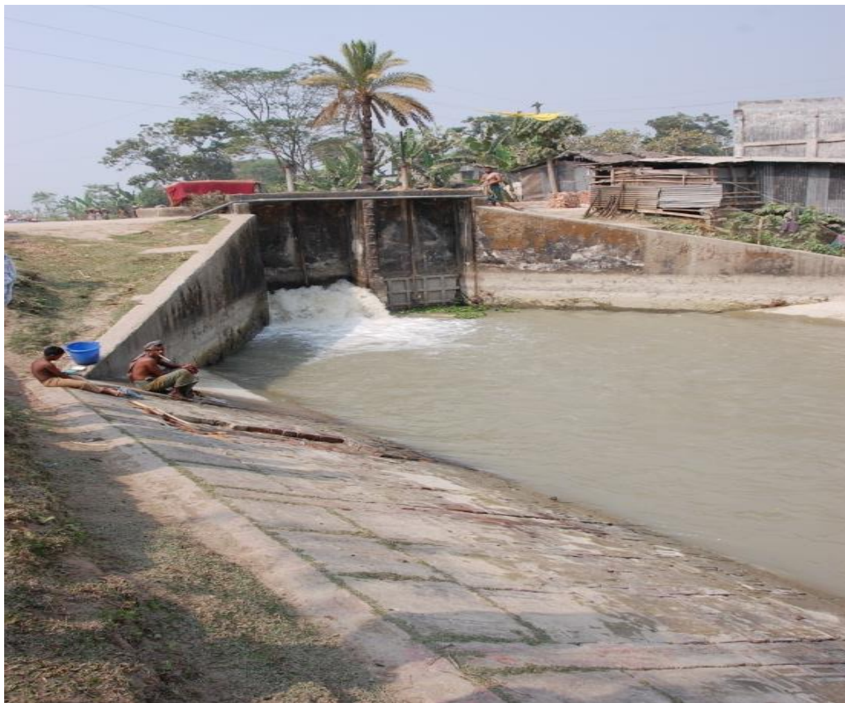
Figure 4. Sluice gate in Amtoli upazila (Source: Field Trip in Barisal region, February 2012)
