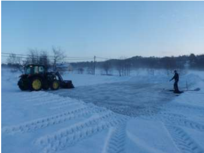
Photo 2. Driving on the 10 cm thick ice layer to remove snow on 25 January. Photo: Trond Pettersen.
