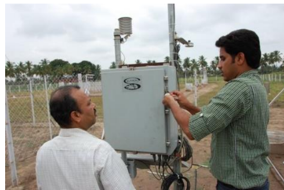
Automatic weather station maintenance
