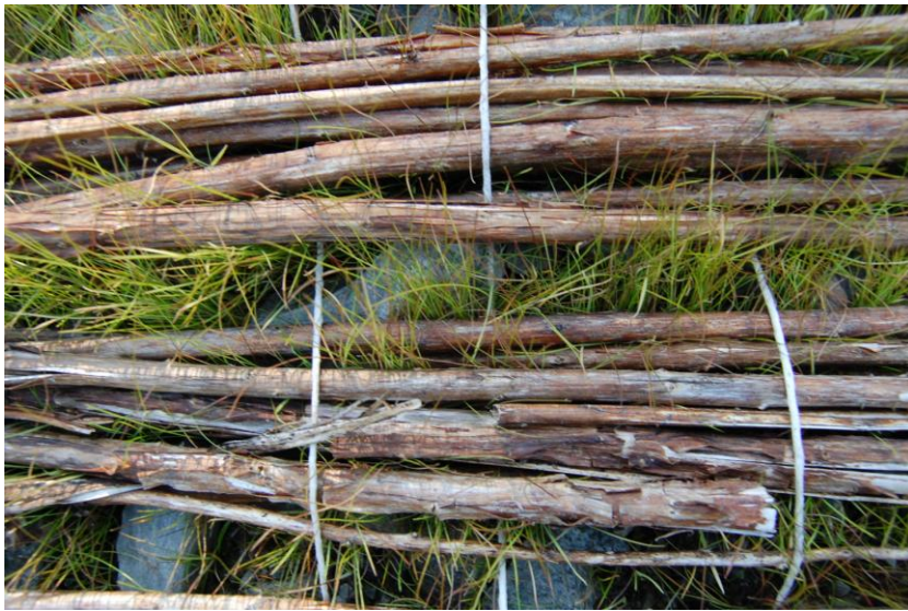
Figure 7. Revegetation trail on a road embankment in Troms County during the first vegetation period using a combination of fireweed mats and native plant material from Flaten field Station (see also Aamlid et al. 2007, this issue). Photo: Christian Uhlig.
