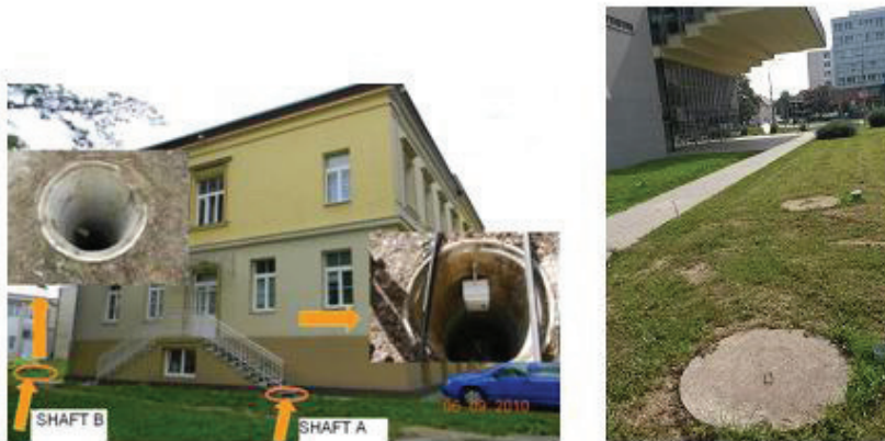
Fig. 6. Infiltration shafts in uUniversity campus in Košice.
