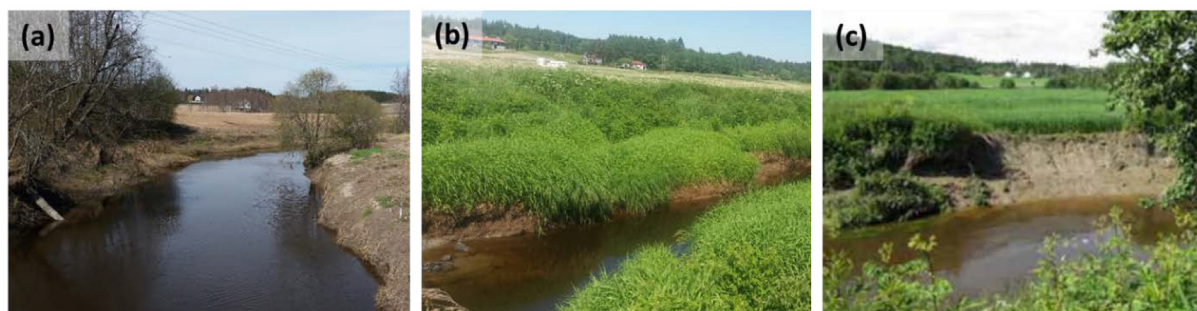
Fig. 1. Examples of observed undercutting processes and associated slope failures in small agricultural catchments in Eastern Norway: (a), Hobøl River and (c) Lier River.
