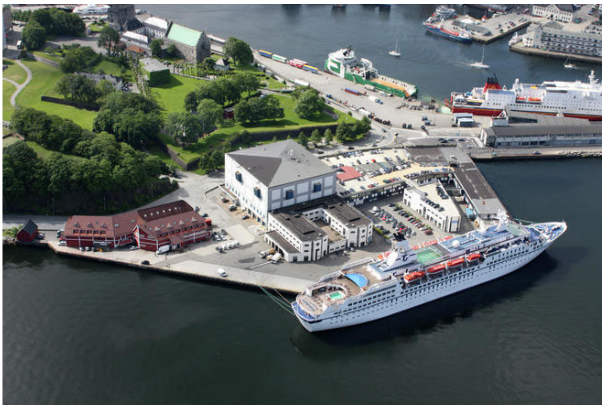
Case study building at Bontelabo. Photo: GC Rieber Eiendom
