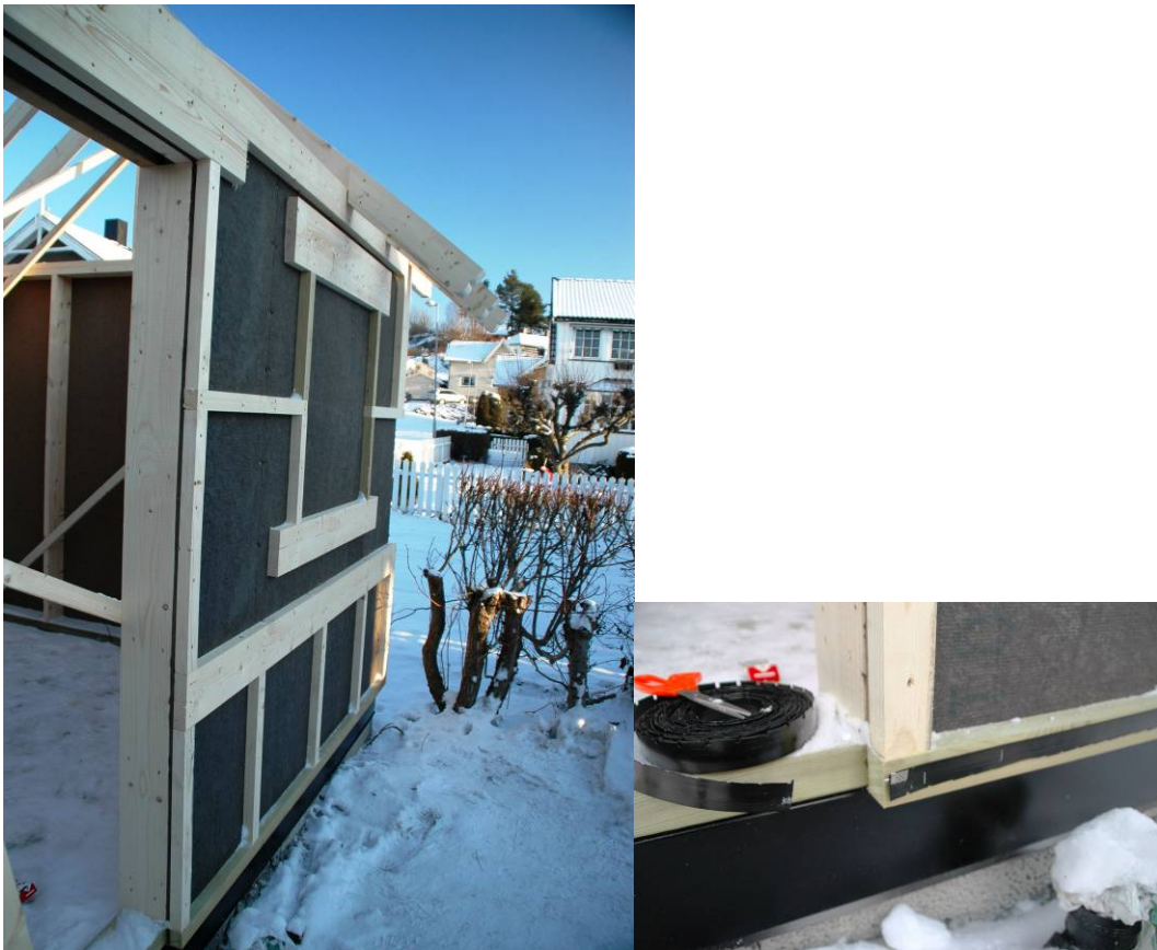
Figure 3: Installation of PLEOT in a building
