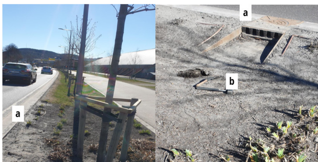
Figure 1. Left picture: the bioretention cell is the area located between the road and the sidewalk. Right picture: inlets specially designed and fitted to the side curb bring road runoff to the bioretention cell. A 13 cm high side curb (a) separates the road from the bioretention cell. Sampling spot in front of an inlet (b).
