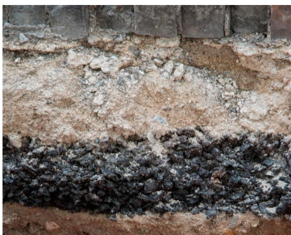
Technosol forseglet under brustein (foto: Franco Ajmone-Marsan (Fabbri et al. 2021)).
