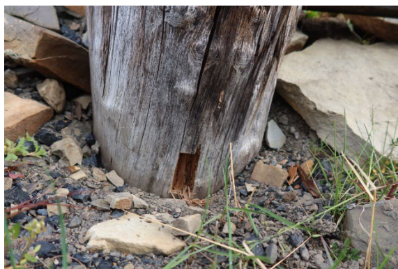
Leg NW, soil contact, after sampling
