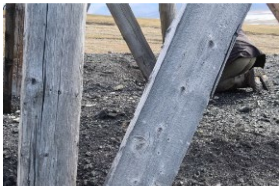
Leg NW, above ground, before sampling
