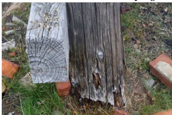
Leg SW, soil contact, before sampling
