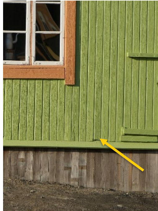
“Museumshytta”, façade facing south-west. Point of awl probing indicated
