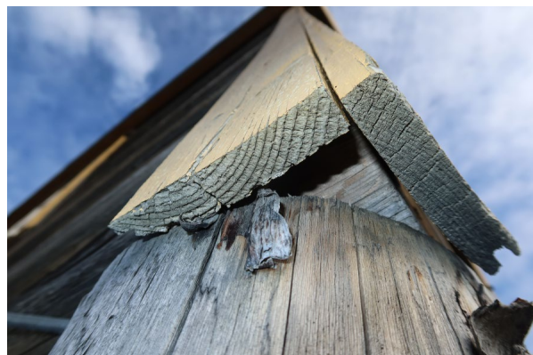
“Direktørboligen”, western facing side. Awl probing performed on end grain of weatherboard beneath main window
