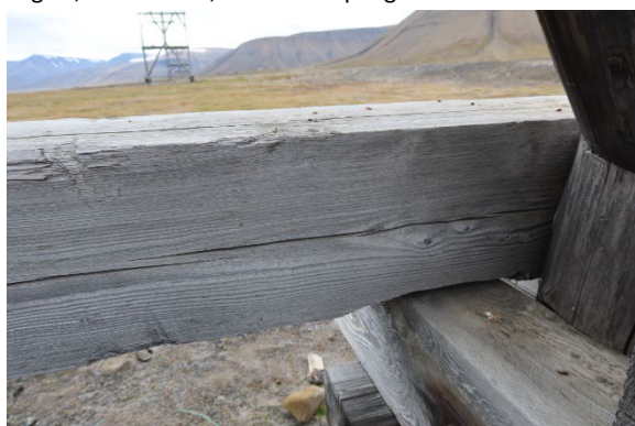
Leg SE, above ground, before sampling
