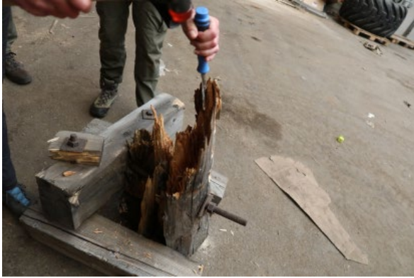
Cable car trestle 87889-16, object 2. Overview
