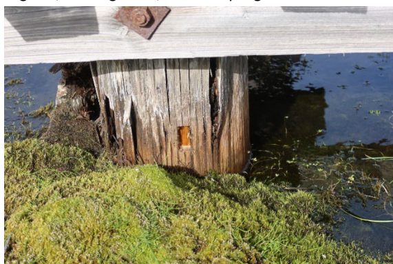
Leg SE, soil contact, after sampling
