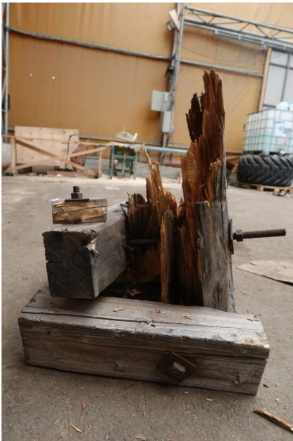
Cable car trestle 87889-16, object 2. Overview
