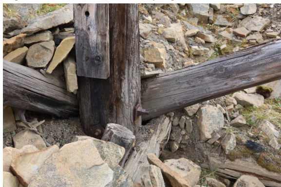
Leg SE, above ground, before sampling
