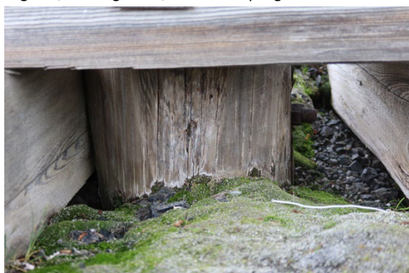
Leg SE, soil contact, before sampling
