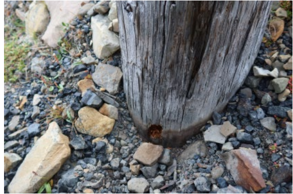
Leg NW, soil contact, after sampling
