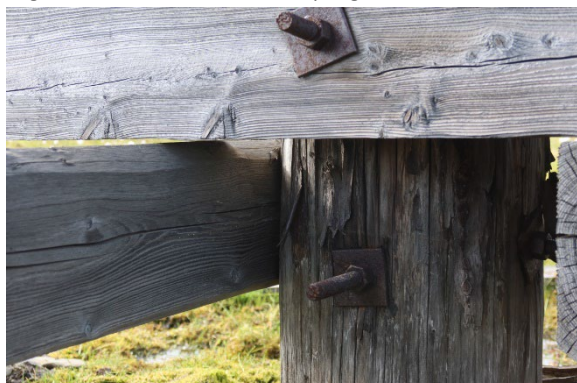
Leg SE, above ground, before sampling
