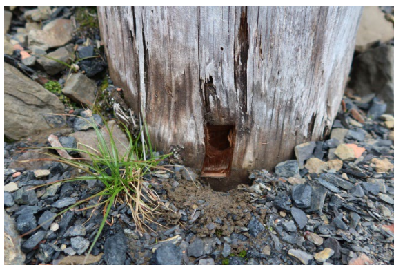
Leg NW, soil contact, after sampling
