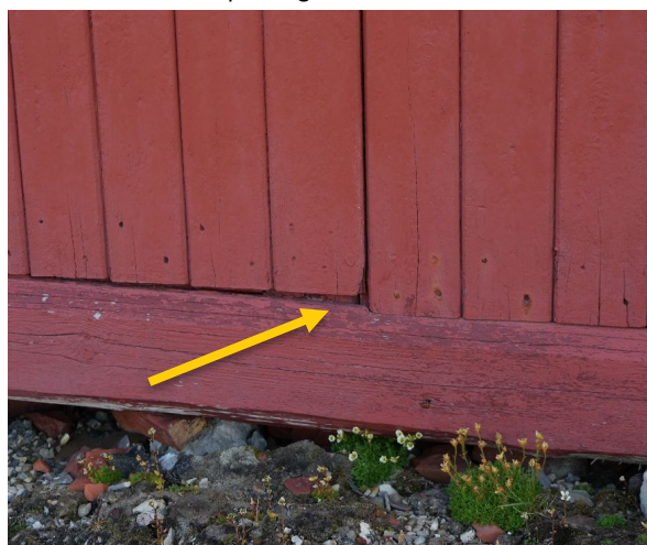
Green Harbour, façade facing north-east. Only façade with window. Points of awl probing indicated
