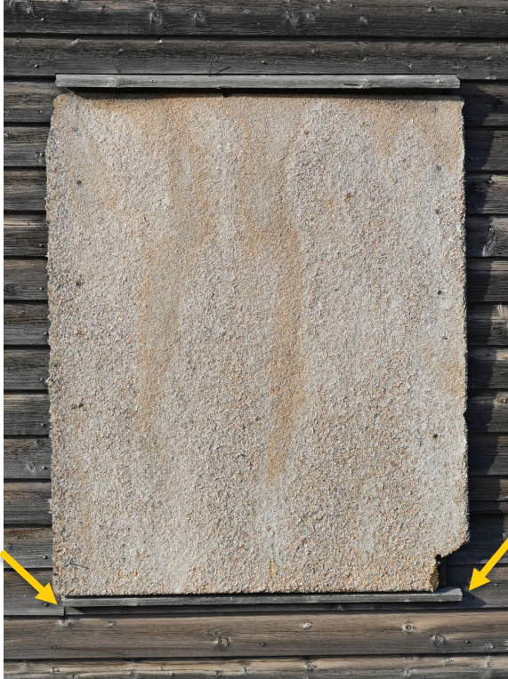
“Sætra”, south-west facing side. Awl probing performed on end grain of weatherboard beneath window.
