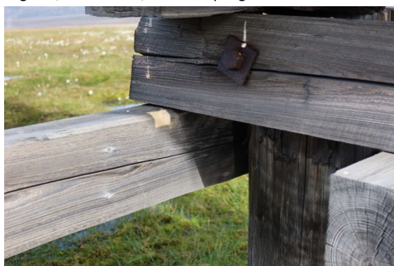
Leg NW, above ground, after sampling
