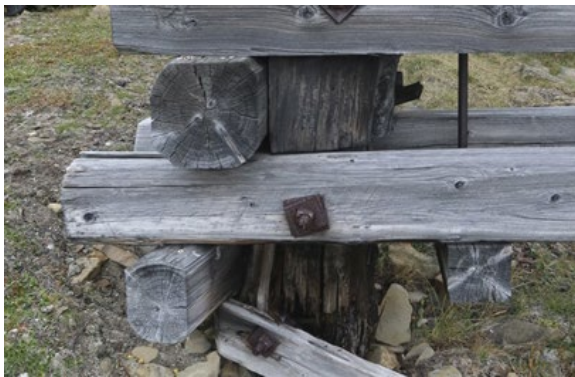
Leg SE, above ground, before sampling
