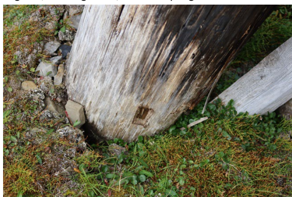
Leg SE, soil contact, after sampling
