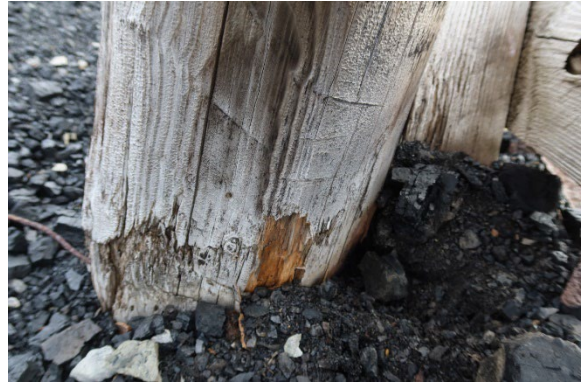
Leg NW, soil contact, after sampling
