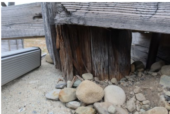
Leg SW, soil contact, before sampling
