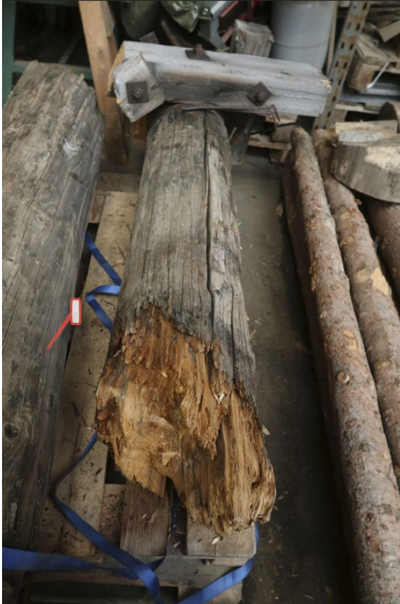
Cable car trestle 87889-16, object 3. Overview
