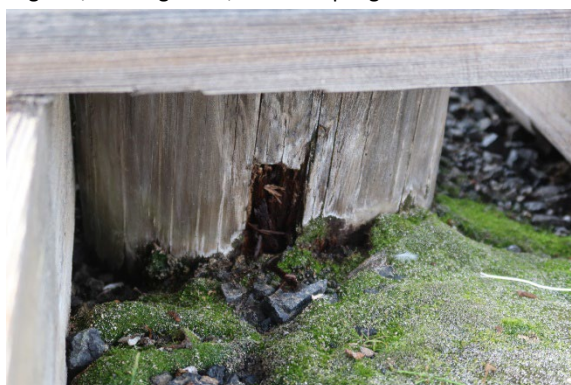
Leg SE, soil contact, after sampling
