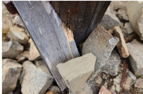
Leg NW, above ground, after sampling
