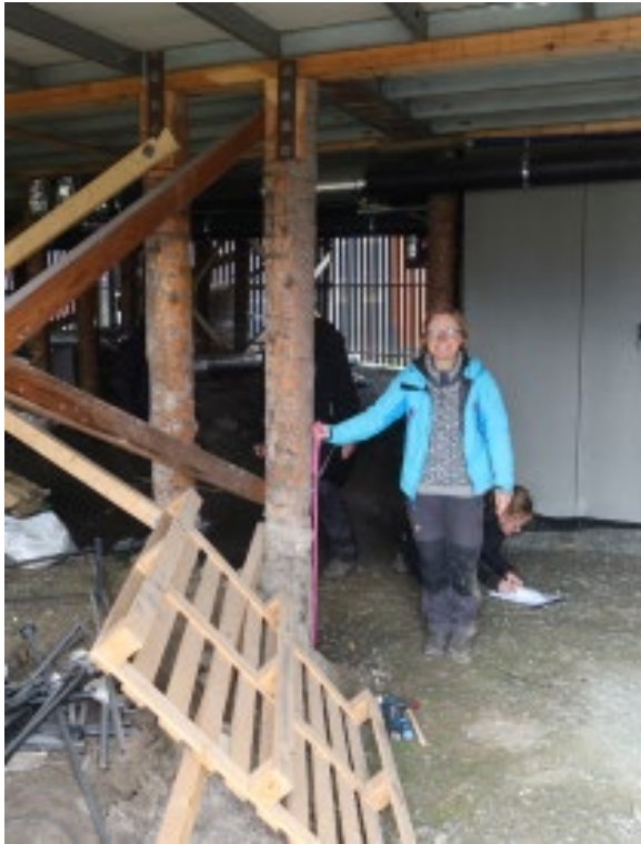
Hotel Radisson Blu, foundation pile SAS2
