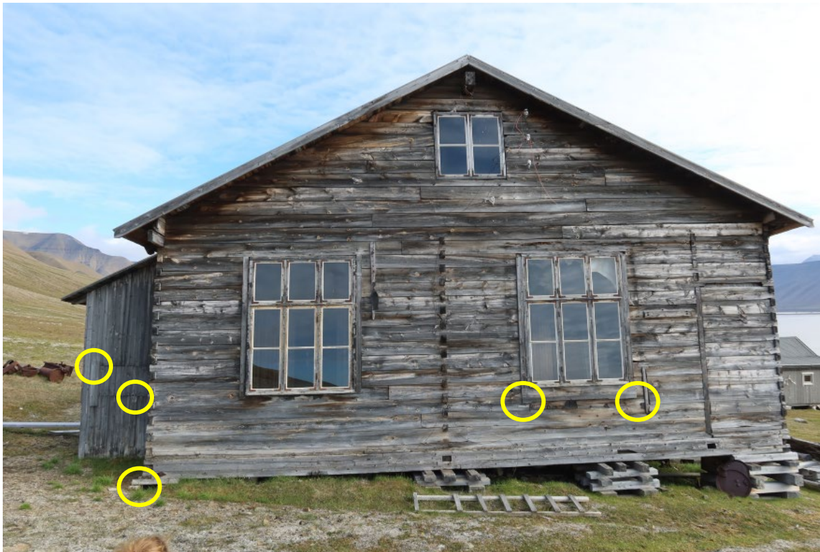
“Boligbrakke”, façade facing west. Points of sampling/drilling/awl probing indicated
