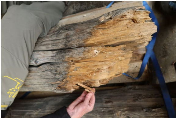
Cable car trestle 87889-16, object 3. Location of sample 3A11
