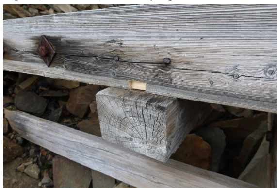
Leg NW, above ground, after sampling
