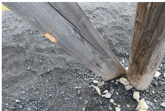
Leg SE, above ground, after sampling
