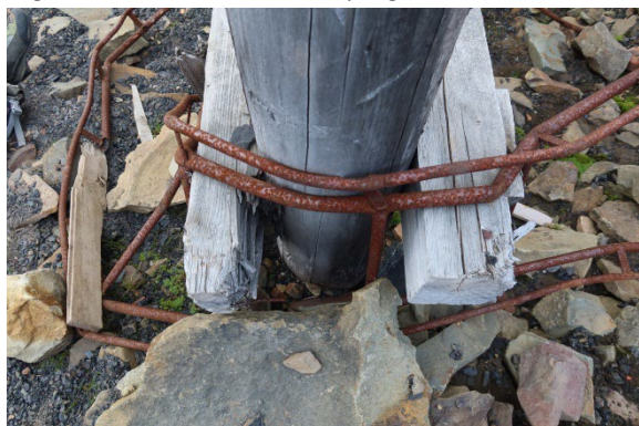
Leg SE, above ground, before sampling
