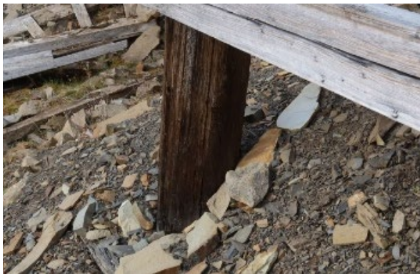
Leg SE, soil contact, before sampling
