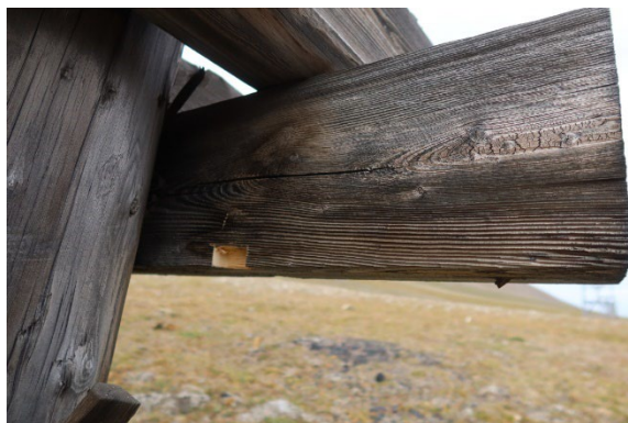
Leg NW, above ground, after sampling
