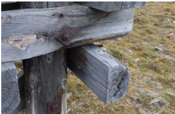
Leg SE, above ground, before sampling
