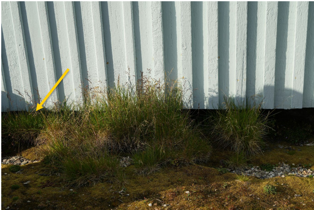
“Mexico”, façade facing south-west. Point of awl probing indicated
