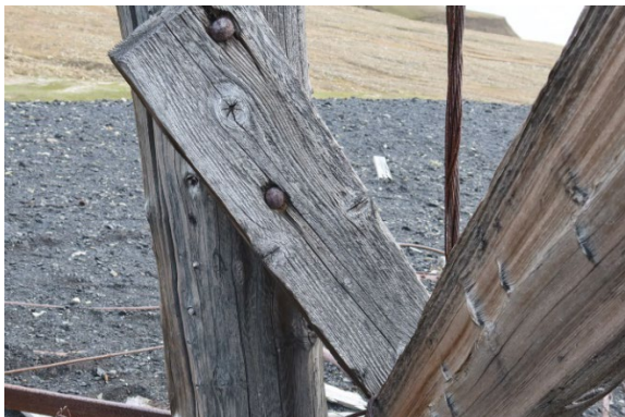
Leg SE, above ground, before sampling
