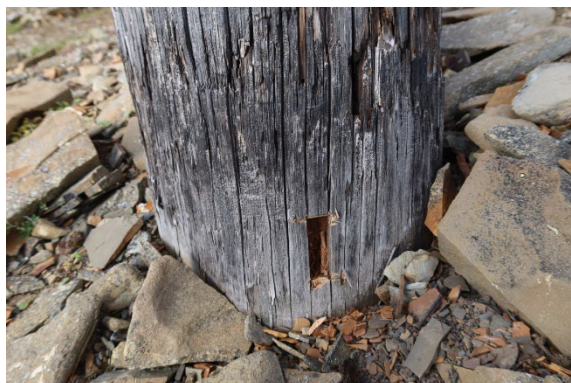
Leg SE, soil contact, after sampling
