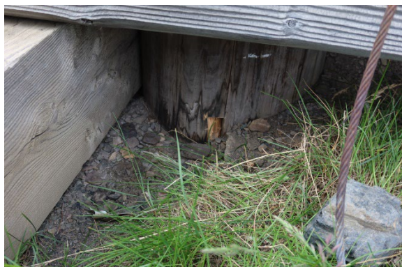
Leg SE, soil contact, after sampling
