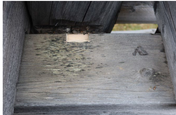
Leg NW, above ground, after sampling
