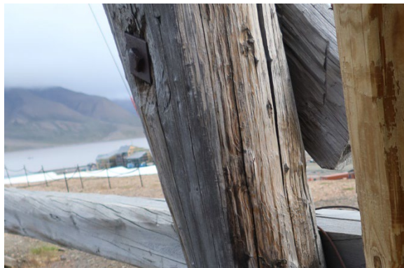
Leg SE, above ground, before sampling
