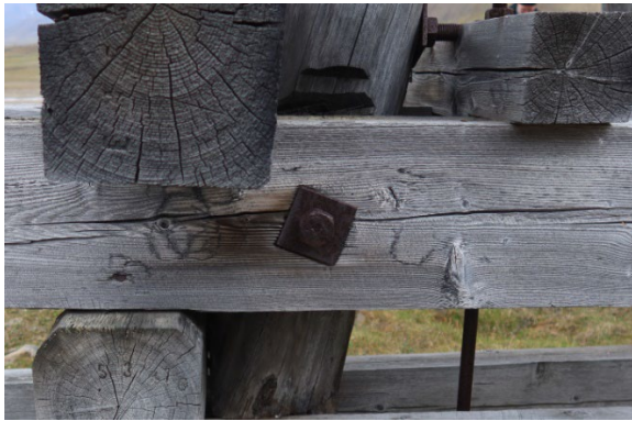
Leg NW, above ground, before sampling
