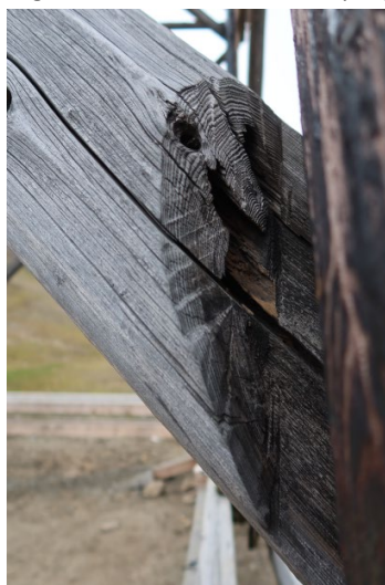
Leg NW, above ground, after sampling
