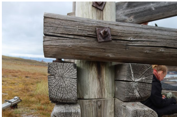
Leg SE, above ground, before sampling
