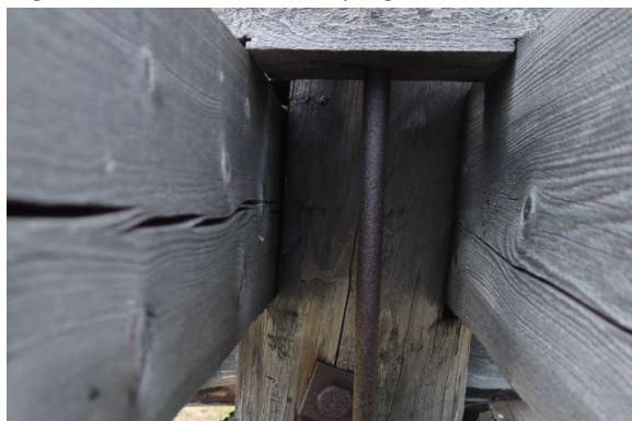
Leg SE, above ground, before sampling
