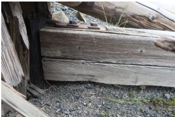
Leg SE, above ground, before sampling
