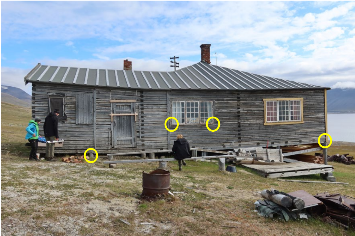
“Direktørboligen”, façade facing west. Points of sampling/drilling/awl probing indicated
