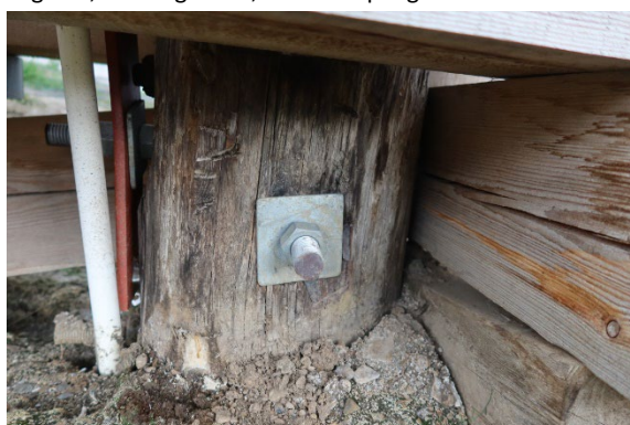
Leg SE, soil contact, after sampling
