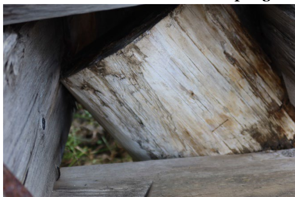
Leg NW, soil contact, before sampling
