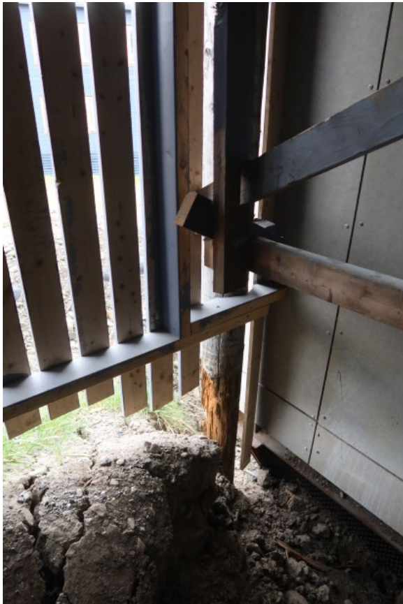
Hotel Radisson Blu, foundation pile SAS1. Overview from the inside
