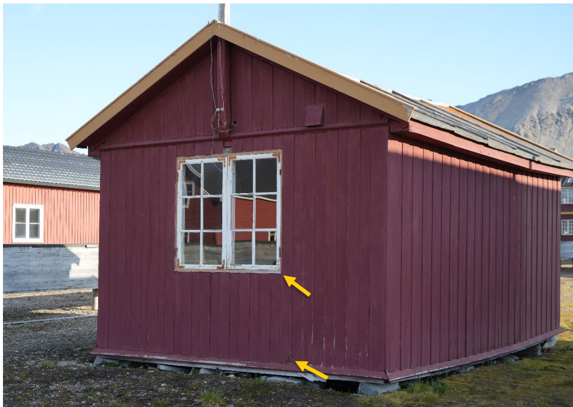
“Museum/Veteranhytta”, façade facing north-east. Only facadewith window. Points of awl probing indicated
