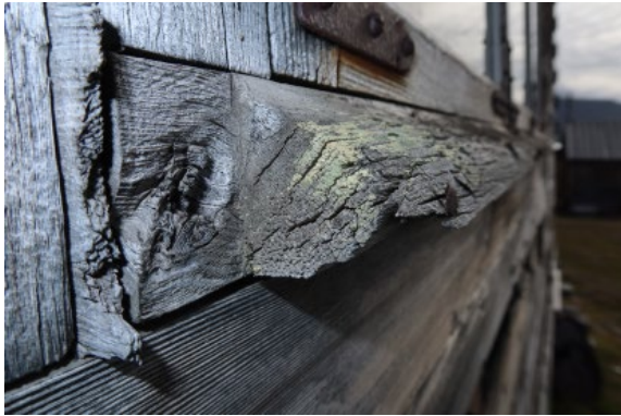
“Boligbrakke”, western facing side. Awl probing performed on end grain of weatherboard beneath southern window
