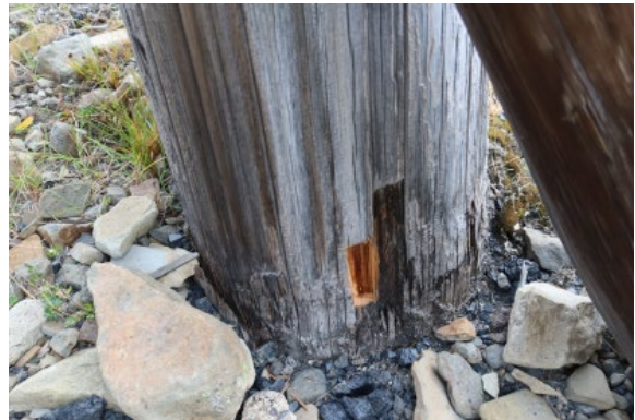
Leg SE, soil contact, after sampling
