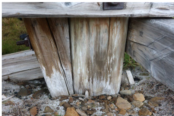
Leg SE, soil contact, before sampling
