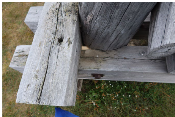
Leg NW, above ground, after sampling
