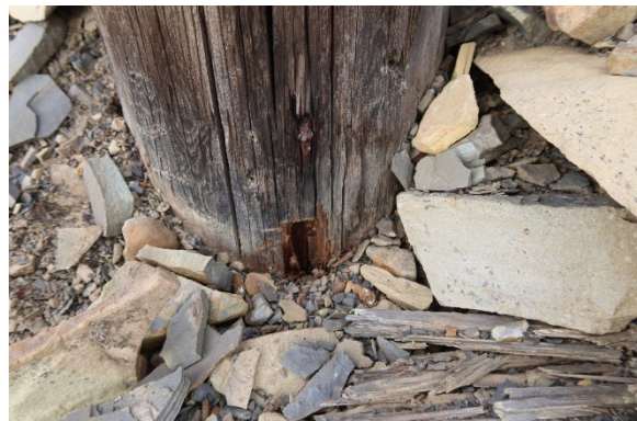
Leg SE, soil contact, after sampling
