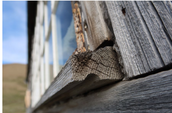
“Direktørboligen”, western facing side. Awl probing performed on end grain of weatherboard beneath main window
