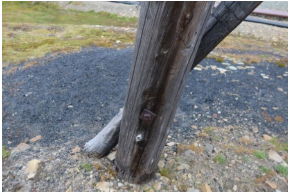
Leg SE, above ground, before sampling
