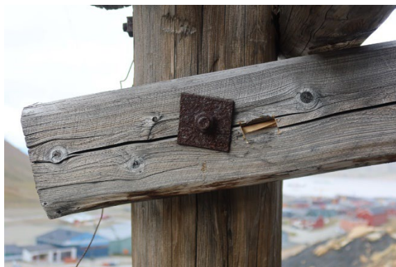
Leg NW, above ground, after sampling
