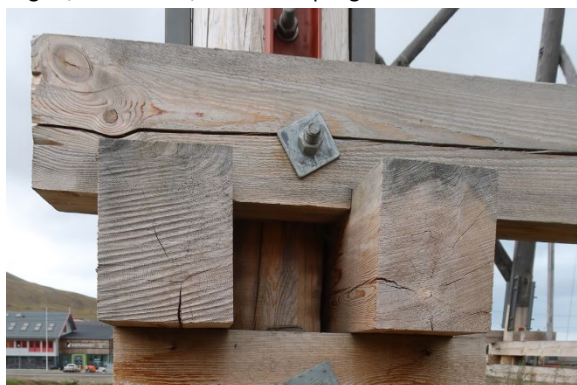
Leg SE, above ground, before sampling
