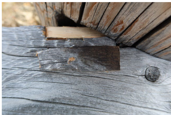
Leg NW, above ground, after sampling
