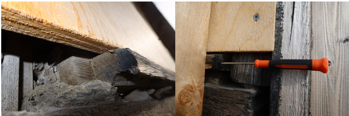
“Telegrafen”, west side. Awl probing in endgrain of weatherboard below window
