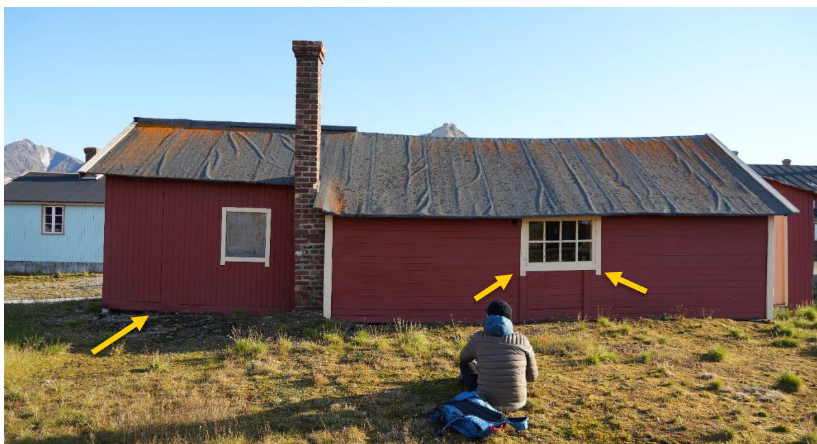
Green Harbour, façade facing north-east. Only façade with window. Points of awl probing indicated
