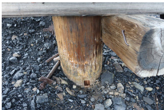
Leg NW, soil contact, after sampling
