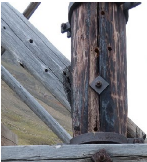
Leg NW, above ground, before sampling
