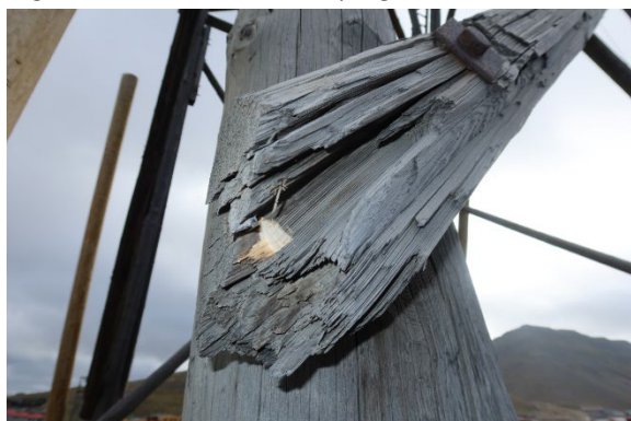
Leg NW, above ground, after sampling
