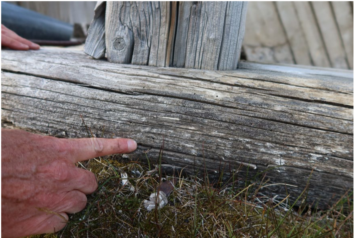
“Taubanestasjonen”, 93041-14. East side. Drilling was done where the finger is pointing
