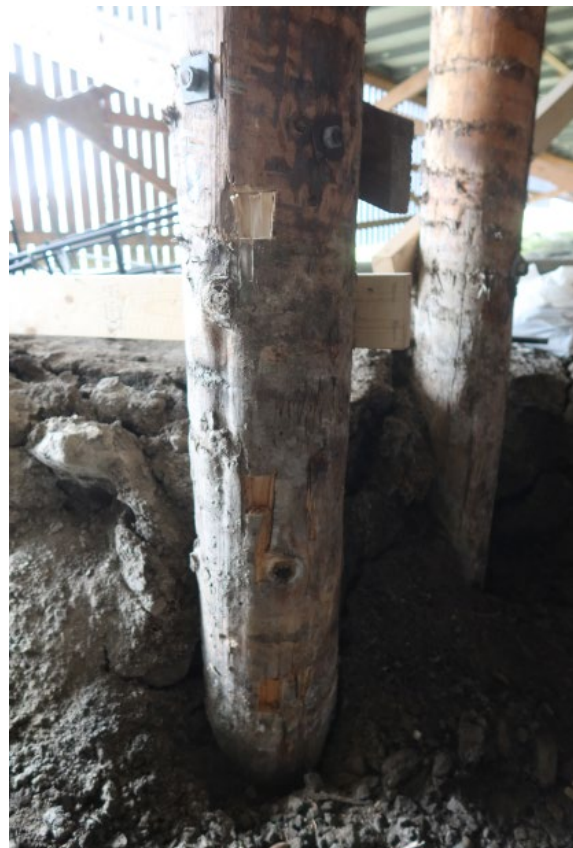
Hotel Radisson Blu, foundation pile SAS2, after sampling
