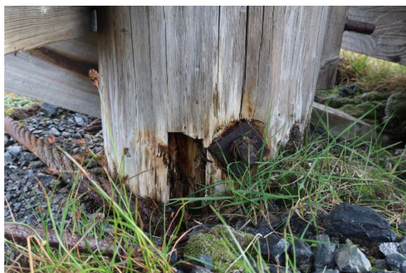
Leg NW, soil contact, after sampling
