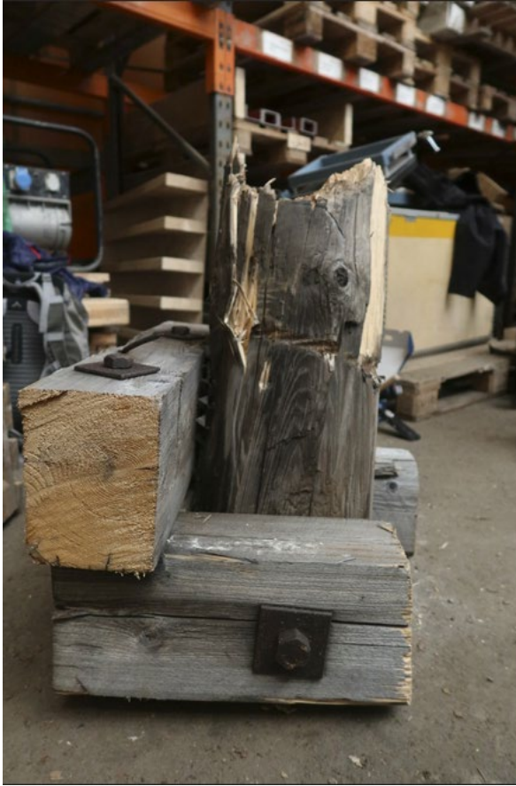
Cable car trestle 87889-16, object 1. Overview
