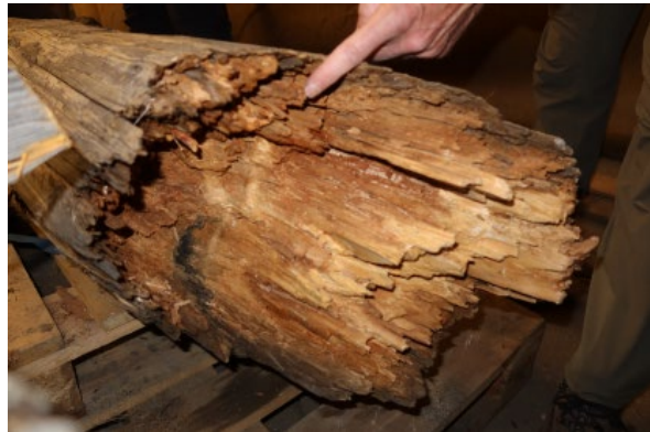
Cable car trestle 87889-16, object 4. Location of sample 4A11
