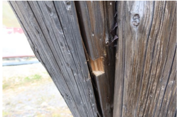
Leg NW, above ground, after sampling
