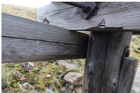
Leg SE, above ground, before sampling
