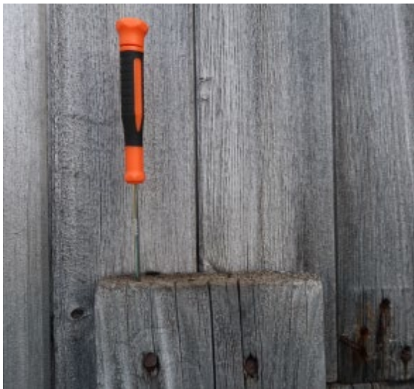
“Boligbrakke”, western facing side. Awl probing performed on end grain of weatherboard beneath southern window
