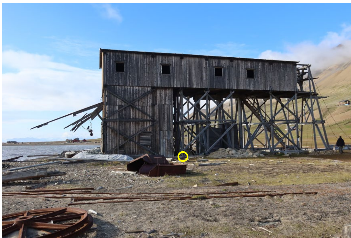
“Taubanestasjonen”, 93041-14. Overview east side. Point of sampling indicated
