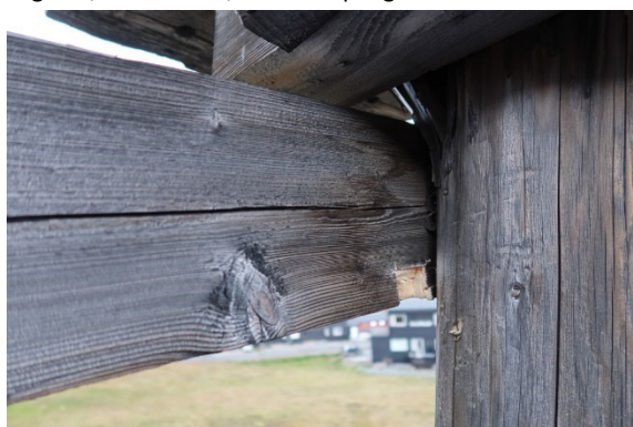
Leg NW, above ground, after sampling
