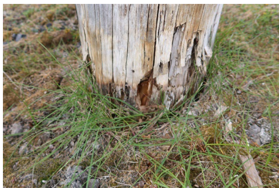
Leg NW, soil contact, after sampling
