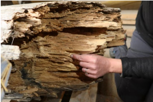
Cable car trestle 87889-16, object 4. Location of sample 4A12
