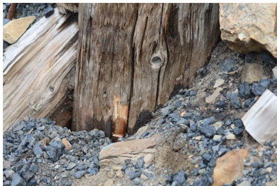
Leg NW, soil contact, after sampling
