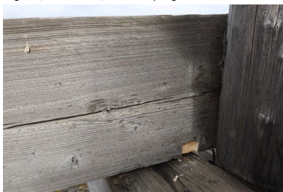
Leg NW, above ground, after sampling
