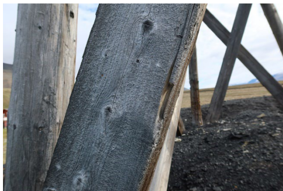
Leg NW, above ground, after sampling
