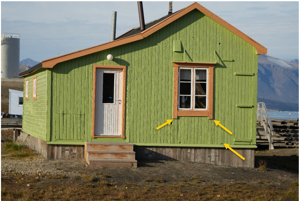
“Museumshytta”, façade facing south-west. Points of awl probing indicated
