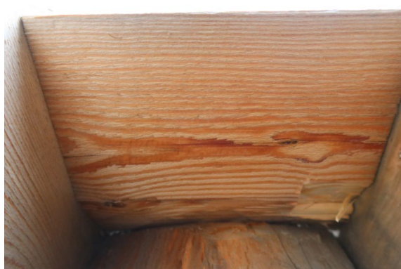
Leg NW, above ground, after sampling
