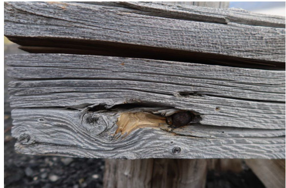
Leg NW, above ground, after sampling
