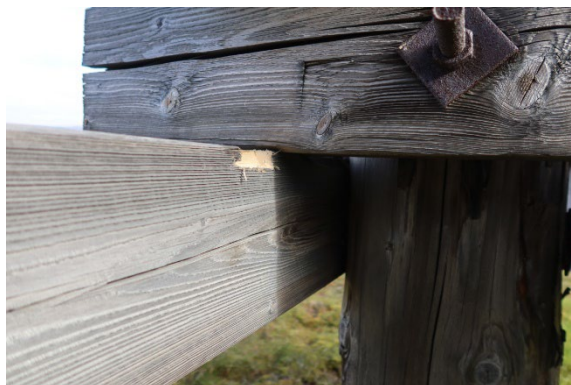
Leg NW, above ground, after sampling
