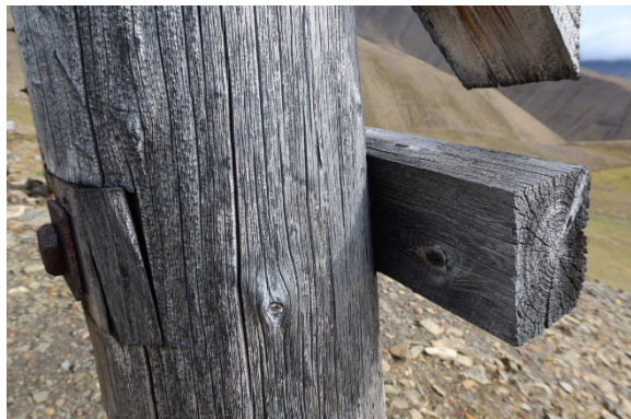
Leg SE, above ground, before sampling
