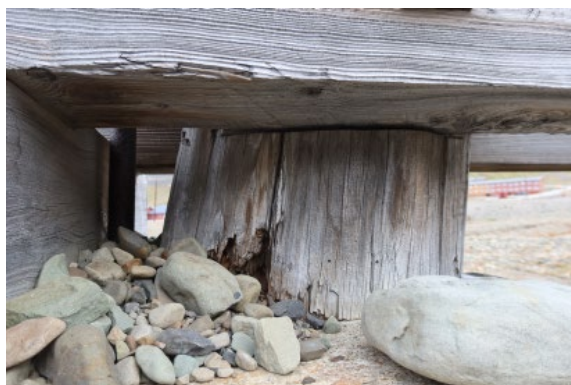
Leg NE, soil contact, after sampling
