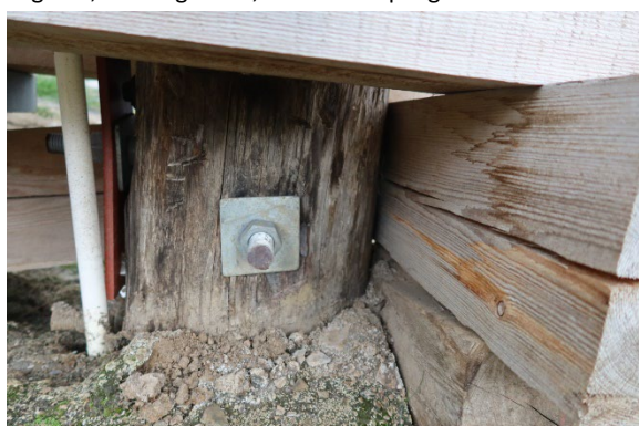
Leg SE, soil contact, before sampling
