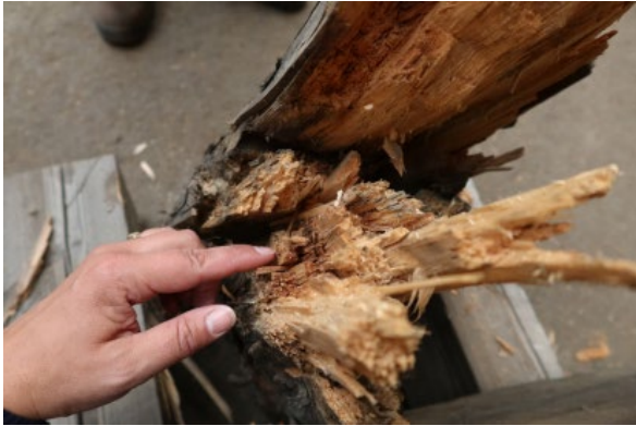
Cable car trestle 87889-16, object 2. Location of sample 2A9
