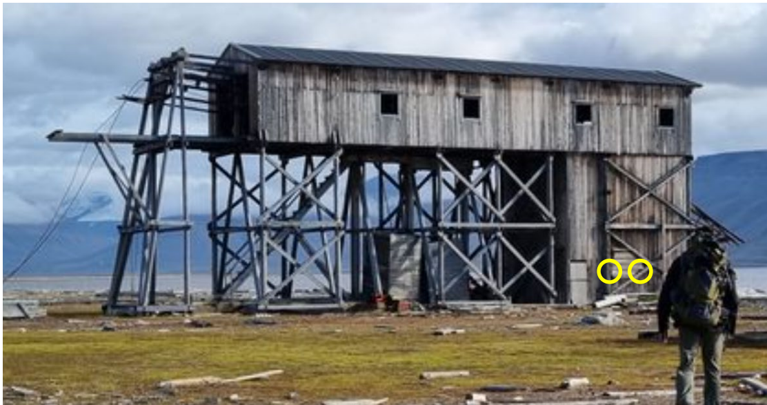
Photos from sampling "Taubanestasjonen", 93041-14. Overview of the west side. Points of awl probing indicated
