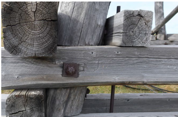
Leg SE, above ground, before sampling
