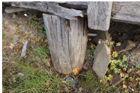
“Direktørboligen”, western facing side. Pile supporting bottom beam, after sampling
