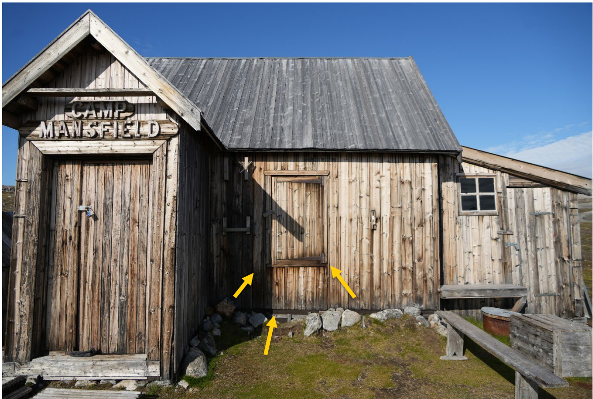
Camp Mansfield, façade facing south. Points of awl probing indicated
