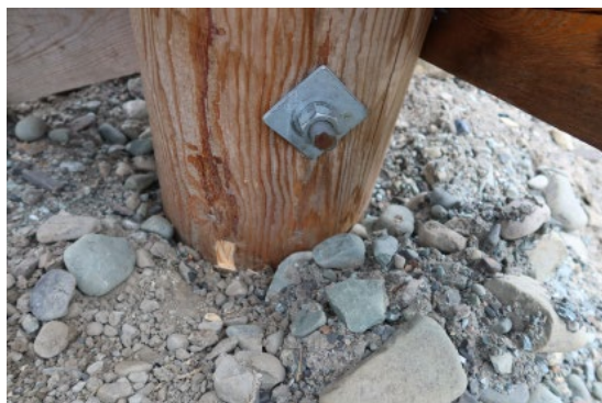
Leg SE, soil contact, after sampling
