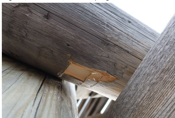
Leg NW, above ground, after sampling
