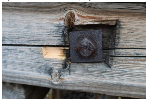
Leg NW, above ground, after sampling
