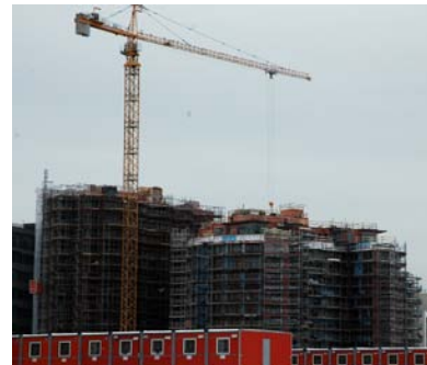
Figur 43. Construction site at Tjuvholmen in Oslo. Photo: GHS.
