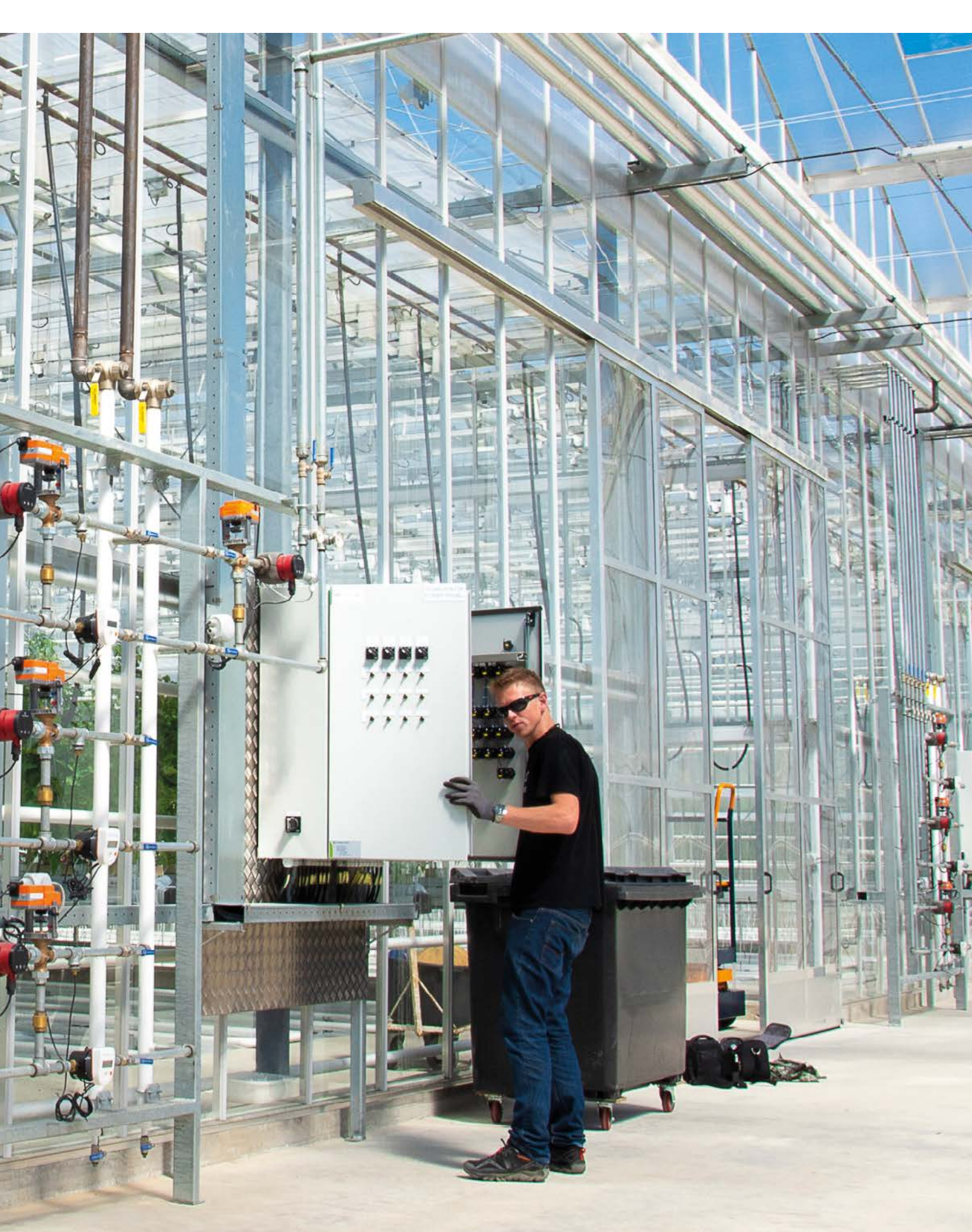
The new greenhouse at the NIBIO Særheim site was opened in September 2018 to enable further growth in the Norwegian greenhouse industry through more research and development cooperation with regional and national research institutes and industry. Særheim now has four experimental greenhouses that cover a total of 2,200 square meters, offering new opportunities for the industry, not only in Rogaland, but across all of Norway. Photo: Erling Fløistad
