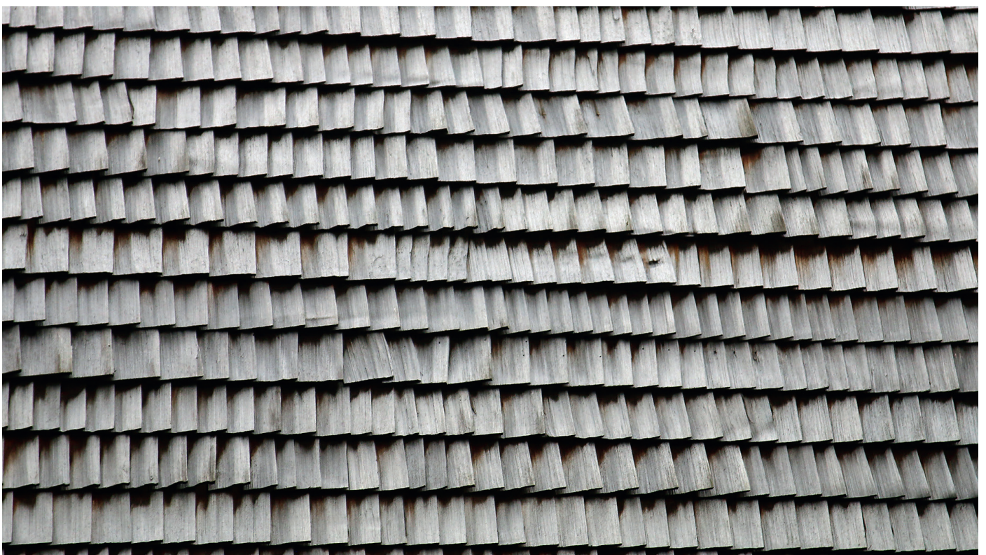
Brueland Kindergarten in Sandnes. Untreated wood shingles cladding, completed in 2012.
