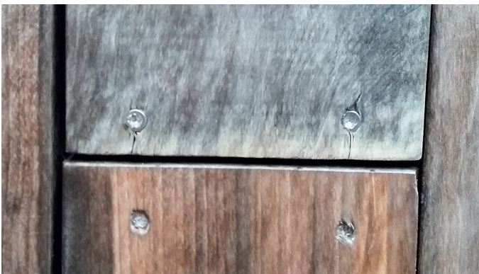
Adequate distance between cladding boards.
