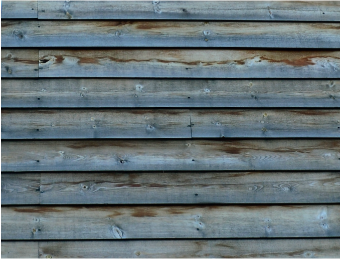
Horizontal cladding of overlapping boards as used in Western Norway.
