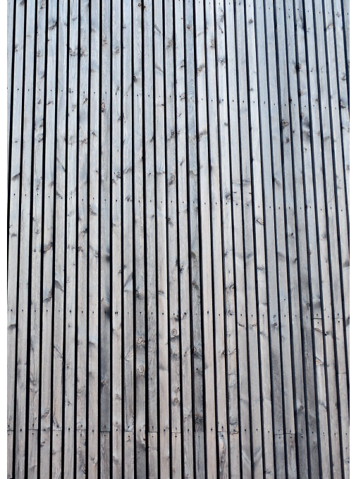
Vertical open cladding.
