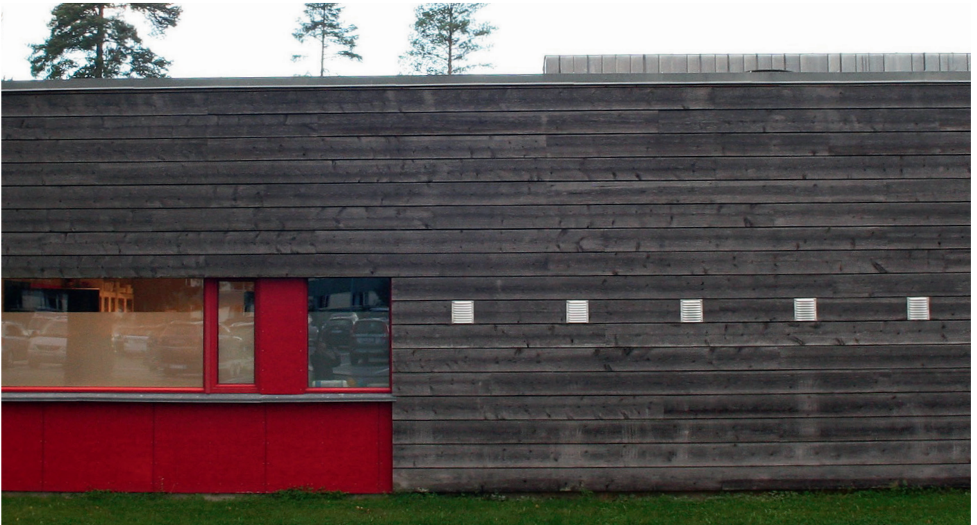
Dry east-facing façade. Lecture building, Sessvollmoen Military Camp.
