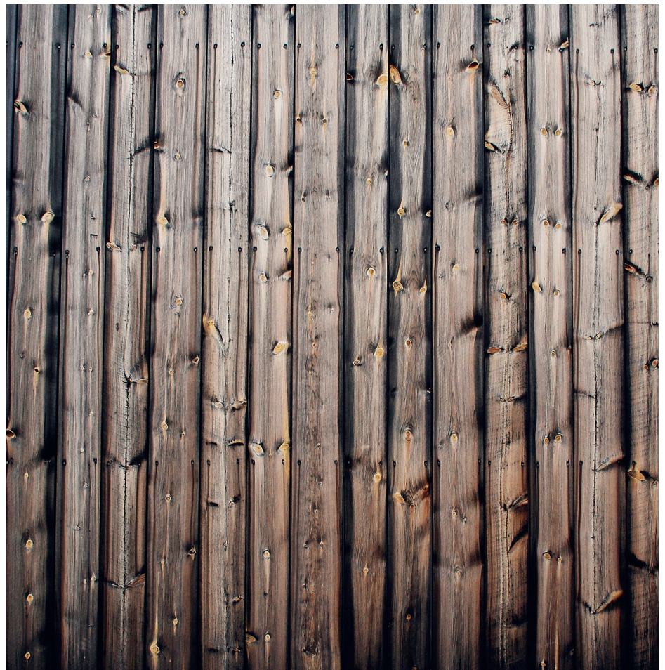
Vertical Scots pine cladding. The cladding boards have a high proportion of heartwood, but some sapwood is present at the edges.
