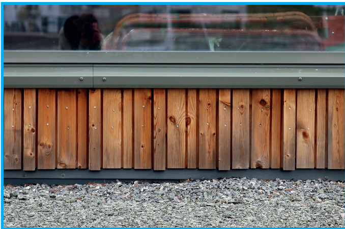
Cladding near the ground that meets gravel
