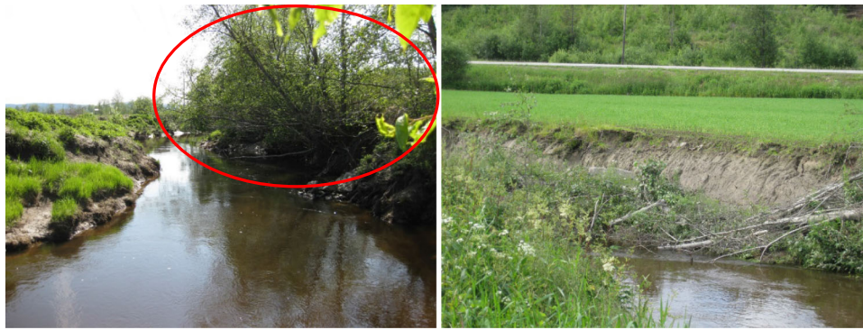
Fig. 5 The importance of trees demonstrated in the Lierelva catchment. A row of trees (in the red circle, left-hand photo) were cut down along the river bank. A few months later, the logs had fallen into the stream, and a steep erosive slope had been formed (right-hand photo). Photos: E. Skarbøvik
