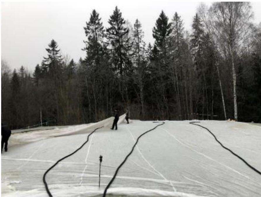
Photo 22. Plastic sheets are pulled over Green 15 (treatment 2) at Asker on 29 Nov. Climate tarp (undercover) and drainage pipes had been laid out on the day before. Sensor sending unit in the foreground. Photo: James Bentley
