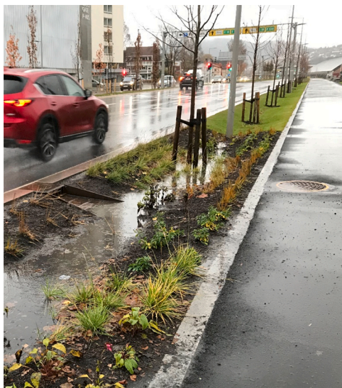
Fig. 2. A rain garden (RG 1) with a drain that directs surface water from the road into the rain gardens during the growing season. In winter, the road water is directed away from the rain gardens to prevent the influx of de-icing salt. The trees are growing in tree planters (not visible on the surface). Photo: Kirstine Laukli.
