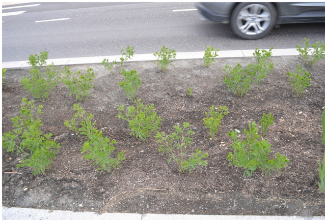
Fig. 5. Grey road dust deposited upon the compost layer is clearly visible, particularly on the roadway side of the rain garden. Photo: Trond Knapp Haraldsen.
