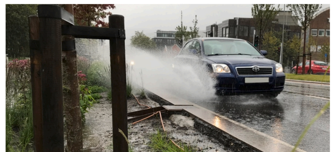
Fig. 4. Splashes from the road in rain garden 1 (RG 1), Bjørnstjerne Bjørnsons Street, Drammen, Norway. Photo: Kirstine Laukli.
