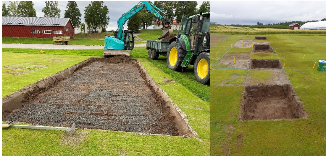
Photo 7: In August 2020, the research green at Apelsvoll was partly reconstructed with the replacement of the rootzone material and new establishment of all creeping bentgrass plots (left) and some plots of colonial and velvet bentgrass (right). Photo: Pia Heltoft
