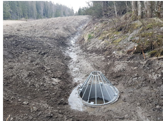
Figure 3.5. (left) Schematic representation of grassed waterways in topographic depression in the field combined with inlets for surface runoff (L. Øygarden) (right) trench for leading excess water from forest into inlets to avoid runoff into agricultural areas (Photo: Ingrid Tenge).
